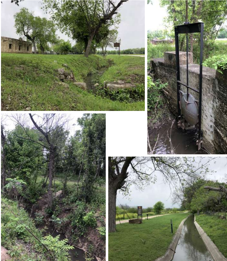
Fig. 4a – San Antonio (Texas), Remnants of a stone compuerta, or sluiceway, in a functioning acequia at mission San Francisco de la Espada (photo, 2024).
