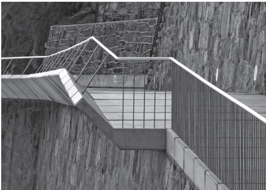
Creus e Carrasco Arquitectos, Harbour Remodelling, Malpica, 2009 (Image from Repertory 07 in Sitografy)
