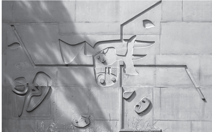
Le Corbusier, Maison de la Culture, Firminy, Bruneaux-Loire, 1959-1967 Bas-relief impressed in the end wall of the building (Photograph Paola Veronica Dell'Aira)
