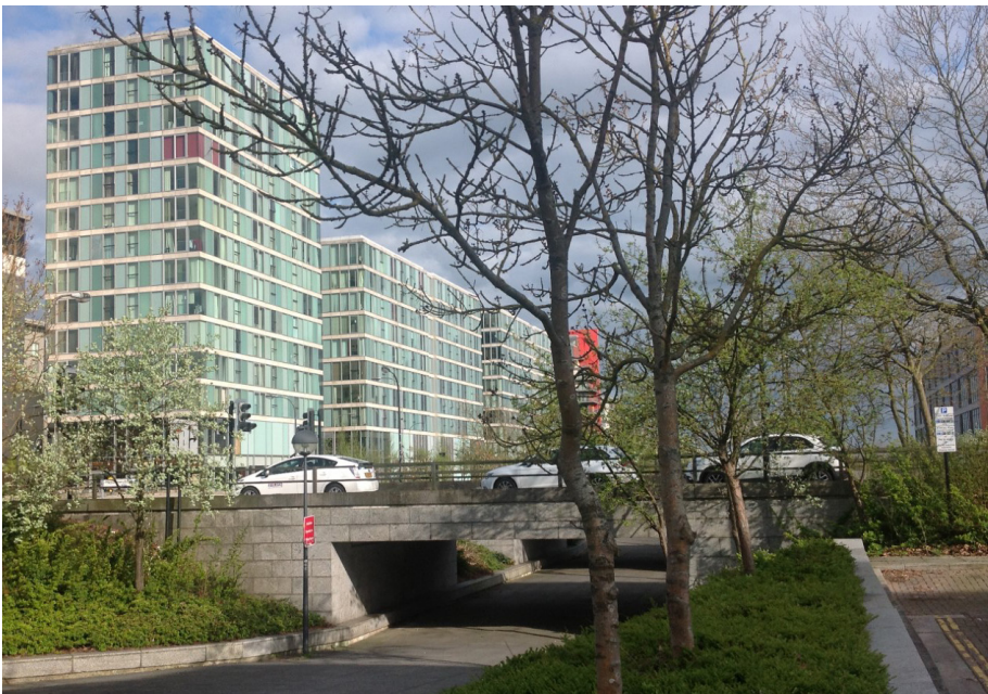
Radburn-influenced separation of motor traffic from pedestrians: an underpass in Milton Keynes (photograph by author; 2016).
